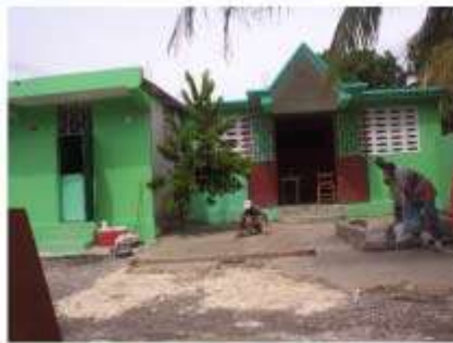
Cement work being done to yard
