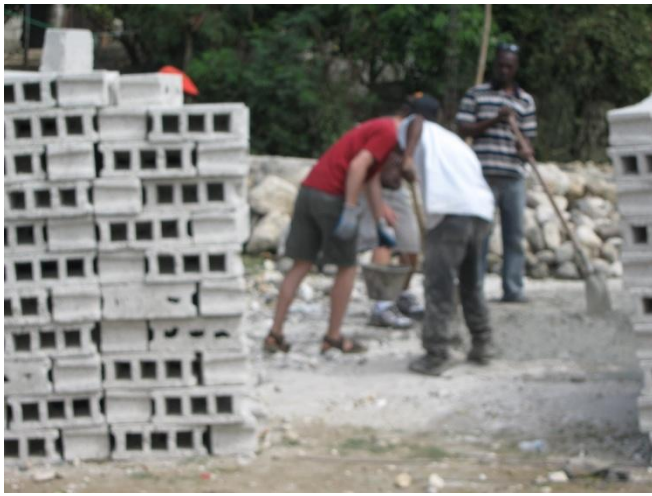
Construction of Security Wall in Rum Village
