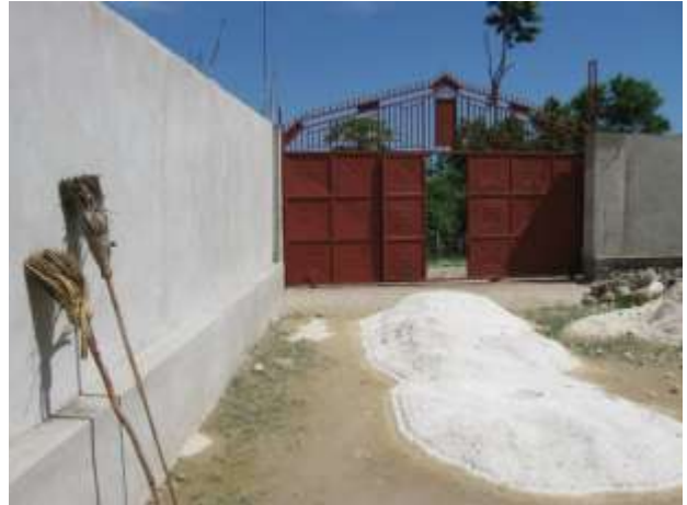
Rebuilt Security Wall
