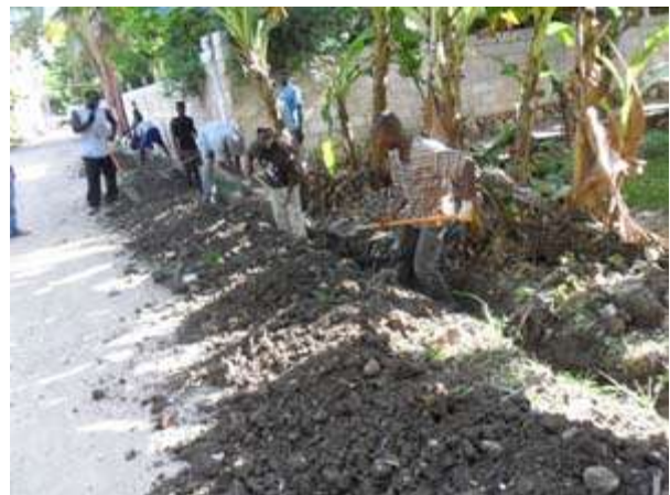
Digging Trenches to Run the Piping
