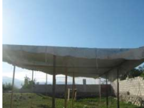
Temporary Church Structure in Rum Village
