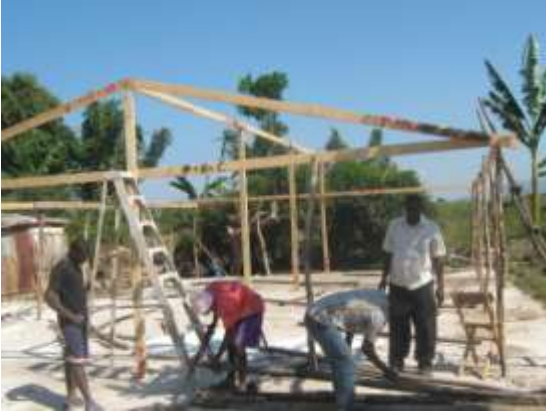
Building Temporary Shelters
