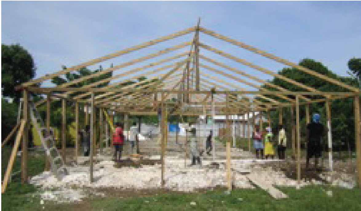
Rebuilding temporary church in TiBrache
